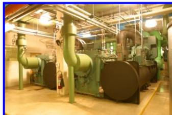
Closed Loop Systems are designed to supply either hot or chilled water to a heat exchanger, and then return the water to the point of origin to repeat the process. Regardless of how the system is designed, the following characteristics apply. Because it is a Closed Loop, no or only minimal losses are expected as there is no evaporation occurring.
